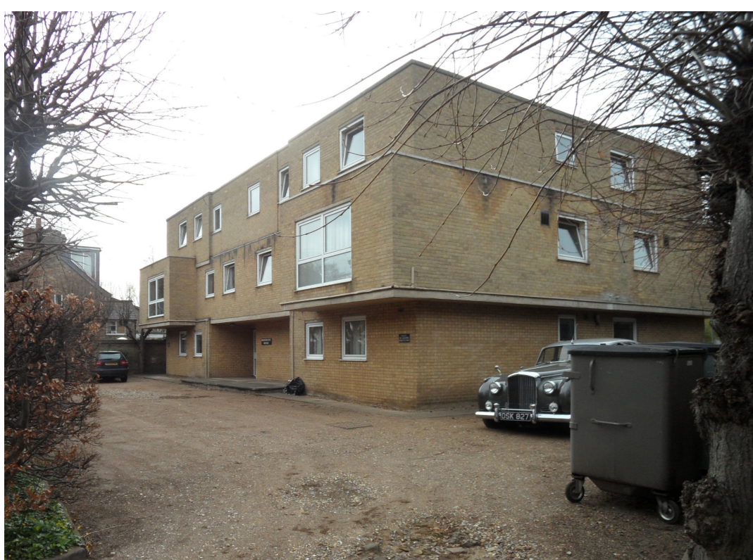
1. View of the existing Whichcote House
