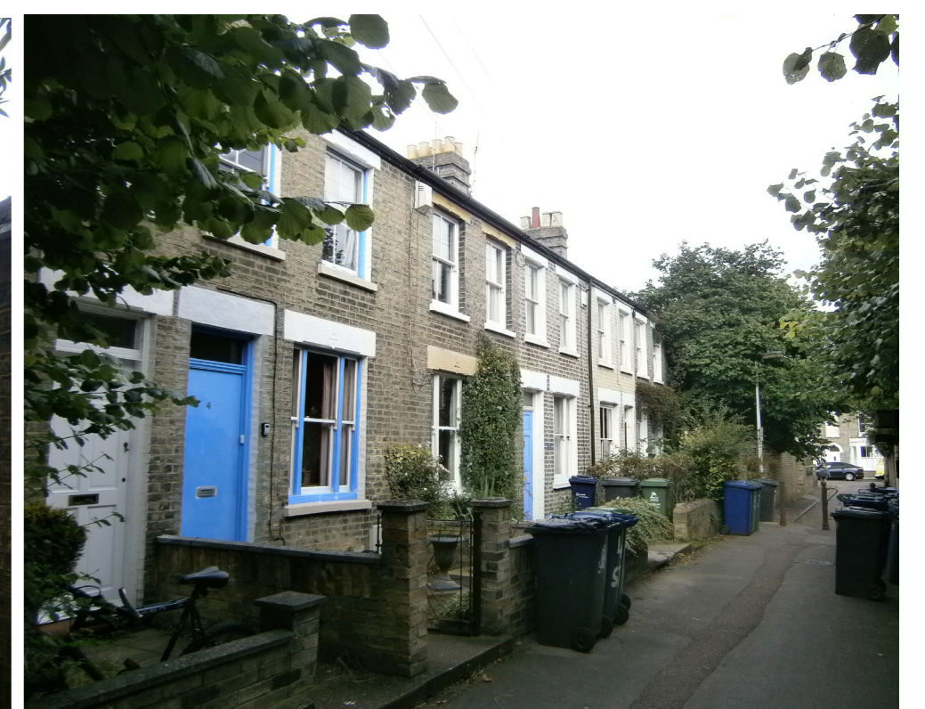
4. Late Victorian terraced houses on Springfield Terrace
