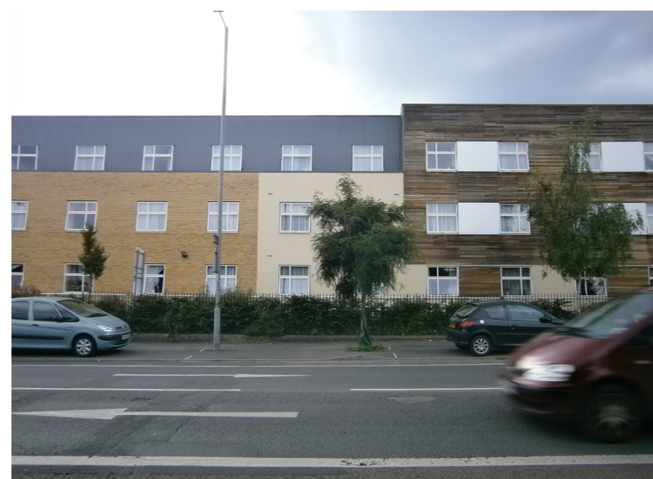
6. Cambridge Manor Care Home opposite the Application Site
